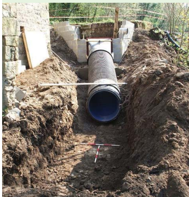
Figure 3.1a/b Burying the pipe ('penstock') carrying the water from the intake to the powerhouse at Alport Mill, Peak District (photos courtesy of Derwent Hydro)
