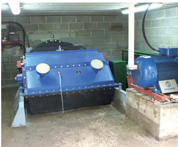
Figure 1.2 The newly installed crossflow turbine at Alport Mill (photo courtesy of Derwent Hydro)
